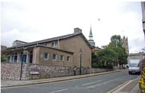
View 14 – looking north along Finewell Street
