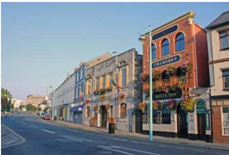
View 12 – looking west along Notte Street
