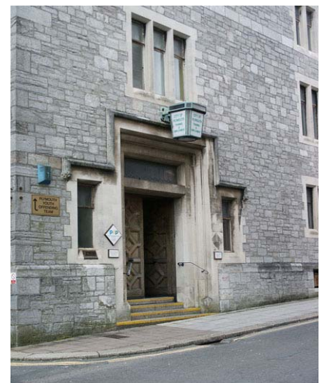
Former police headquarters, rear of Guildhall, Catherine Street
