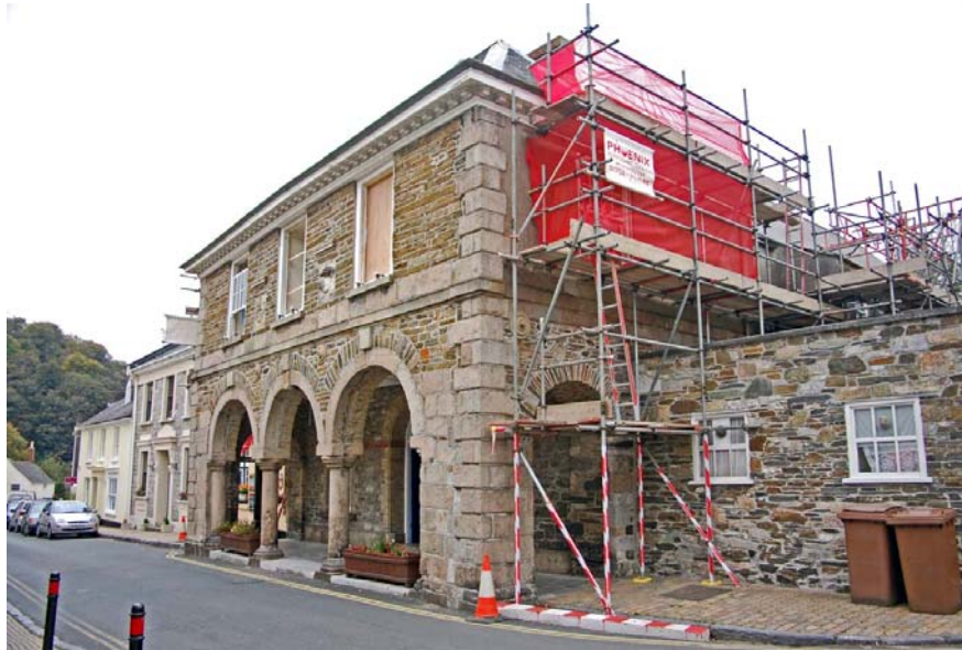
Repairs to Guildhall 2007
