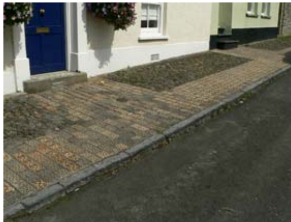
Candy Tile paving in Fore Street
