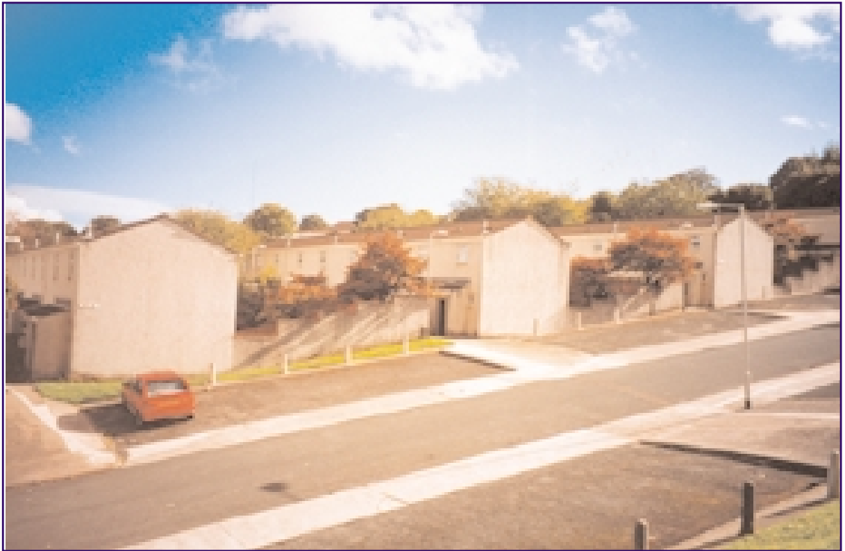
Tailyour Road, Crownhill, ex-MoD properties prior to redevelopment
