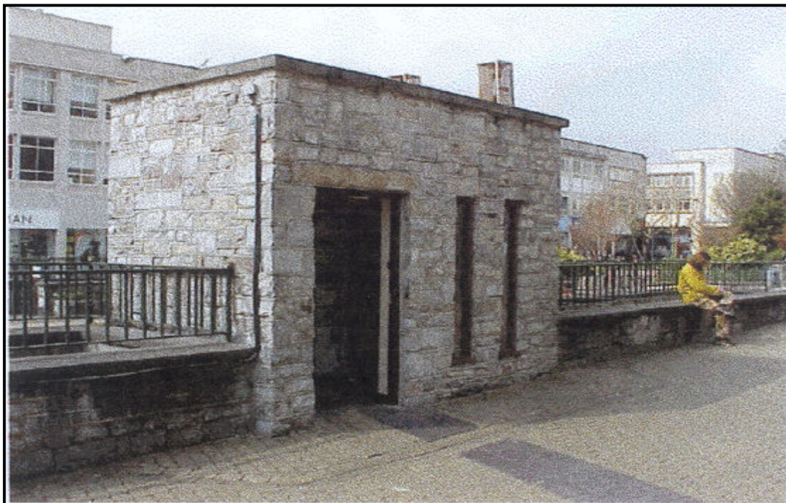
Figure 1.1: Automatic Urban Monitoring Site in Armada Way, Plymouth
