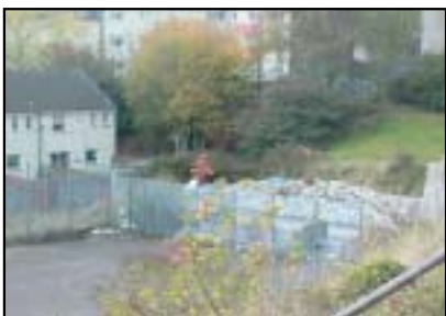
5. View looking west onto demolished buildings
