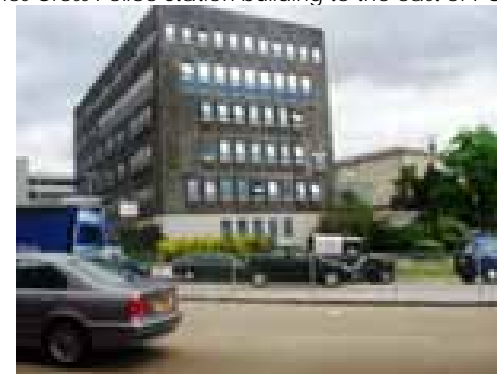
Charles Cross Police Station building to the east of PCAD site
