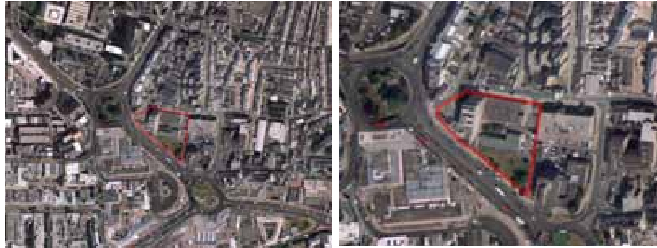
Aerial views of main PCAD site
