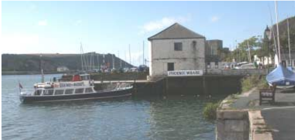
Phoenix Wharf Landing Stage
