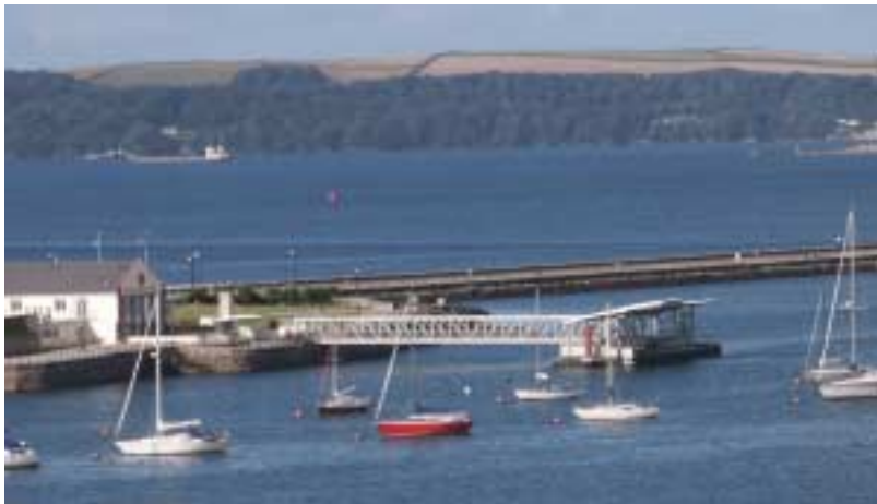
Mount Batten Landing Stage
