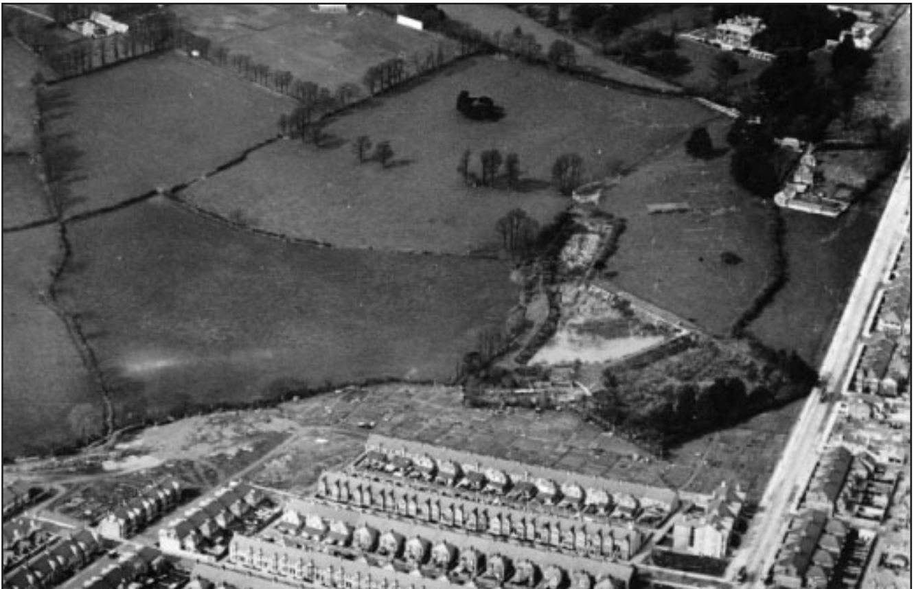
Late 1920s aerial view of Pounds House
